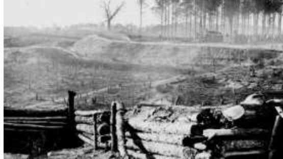
Bermuda hundred earthworks
